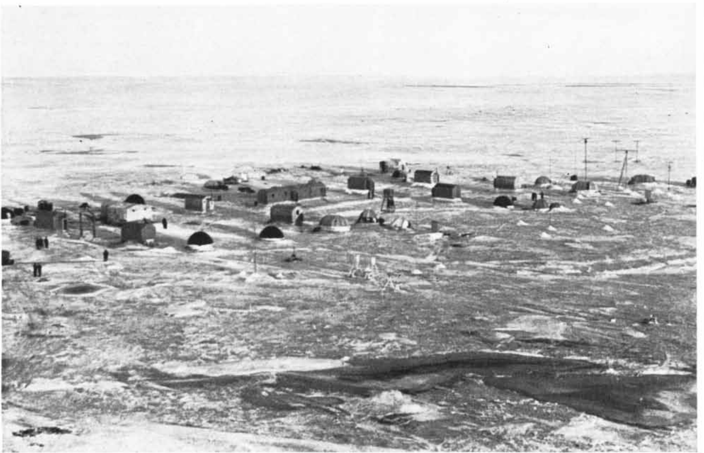
ICE ISLAND NORTH POLE VI , a Soviet observatory established on the drifting ice, began a 700-mile journey in 1956 and ended it 27 months later. Hemispherical structures are laboratory tents; rectangular ones, living quarters. At right are radio antennas.
