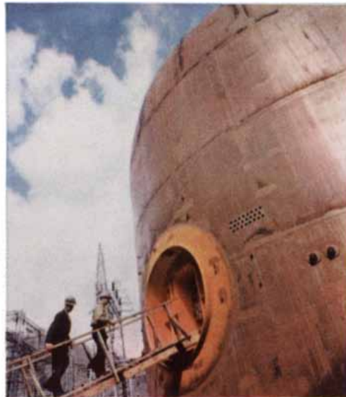
Westinghouse Engineers, after design, follow through on construction of reactor plants such as this 5,000 kilowatt plant being built at Saxton, Pa., for the Saxton Experimental Corporation. This new reactor will be used with an existing turbine generator at the Pennsylvania Electric Company site.
