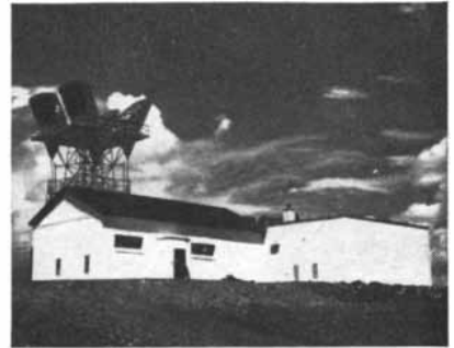
It was completing the development of a new “heavy route” Long Distance microwave system capable of handling over 11,000 two-way conversations at once.
