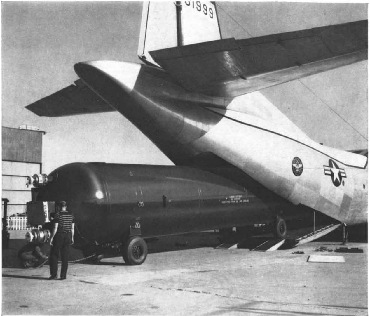
Airborne liquid oxygen tank is loaded aboard a U.S. Air Force Douglas C-133 for flyaway delivery to Vandenberg Air Force Base, California, to become part of the ground support system for the Thor missile.
