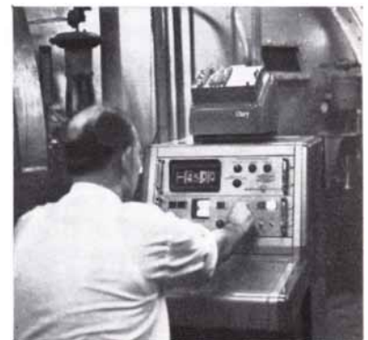
SPACE MEDICINE RESEARCH. In simulated space environment testing, this NLS V34 digital voltmeter is part of a system which detects and records minute changes in body weight, a key factor in determining physiological strain. The unique "No Needless Nines" logic of the V34 permits measurements at pre-selected time intervals with an accuracy of \pm 3 grams within a range of \pm 4,500 grams. AMF's Mechanics Research Division developed the overall system under direction of the Air Force's Aeronautic Systems Division at Wright-Patterson AFB in Ohio.
