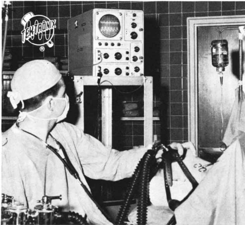
Anesthesiologist observing blood pressure and ECG waveforms of patient during surgery—on full 8-centimeter by 10-centimeter display area of Tektronix Type 502 Oscilloscope—at North Carolina Memorial Hospital, Chapel Hill, North Carolina.
