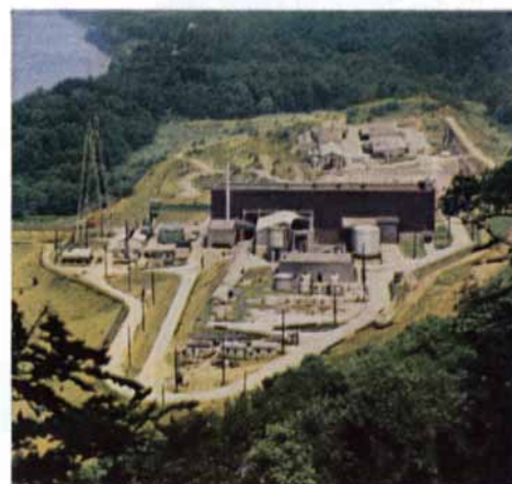
SHIPPINGPORT, PA. Plant of Duquesne Light Co., the nation's first nuclear powered central station. Reactor designed by Westinghouse in cooperation with Naval Reactors Branch of the AEC.
