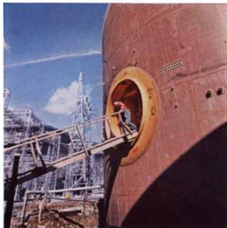
SAXTON, PA. An experimental water reactor to be used with an existing turbine-generator of the Pennsylvania Electric Company.
