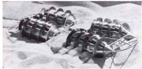
Moon-Roving Concept —This early model moon rover utilizes the principle of the Archimedes screw . . . and is just one of a number of vehicle types under study for known lunar conditions.
