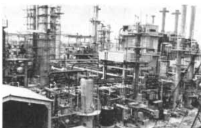
Plant yields were optimized and safe operating levels were set for this new naphthalene plant at Sun's Toledo Refinery by process simulation using an analog computer.
