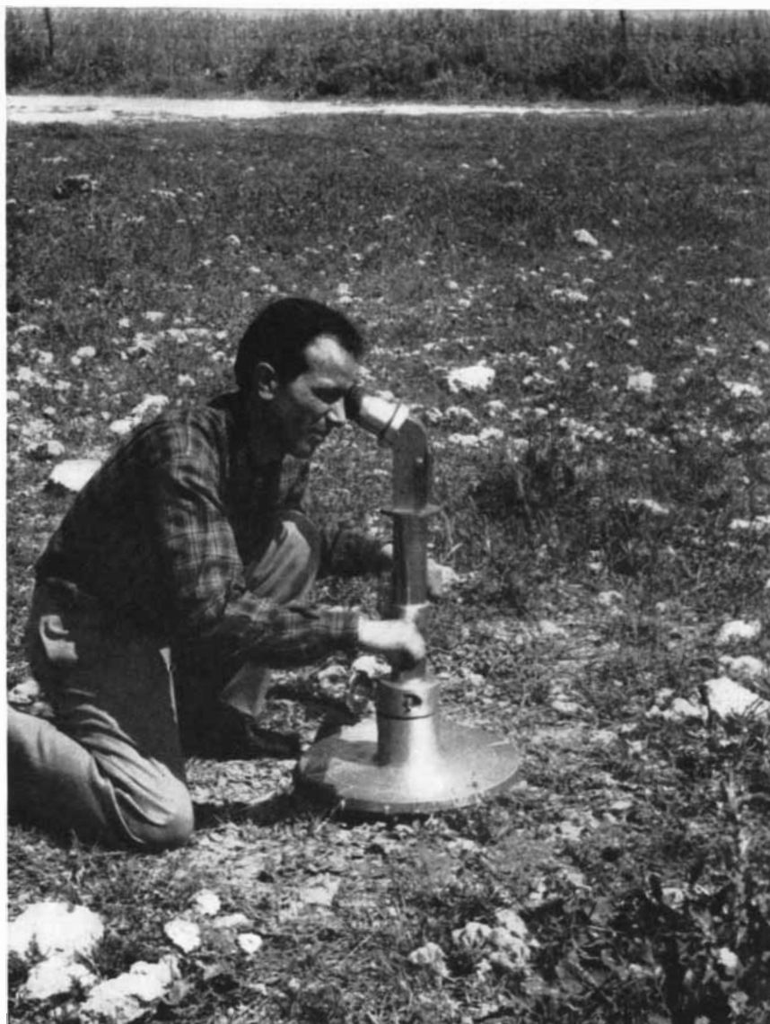
PERISCOPE is used to look into a tomb located with the potentiometer. The funds and technical assistance for this work have been provided by the Lerici Foundation of Milan.
