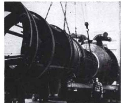
Baldwin-Lima-Hamilton built evaporator bundle being inserted in shell contains a honeycomb network of Anaconda core tube, built to withstand temperatures ranging from 304 to 895°F.
