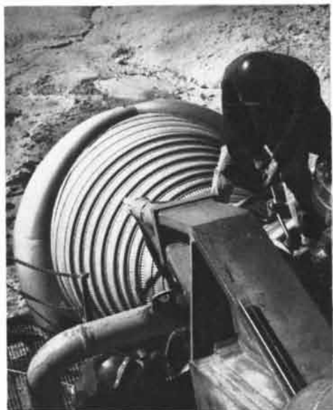
Workmen complete assembly of the F-1 thrust chamber, which has thin-walled tubing brazed with a palladium containing alloy. This chamber later produced the highest thrust ever achieved—1,640,000 pounds on April 6, 1961.
