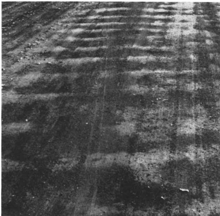
MODERATE CORRUGATIONS are seen in this photograph made in the Australian state of Victoria. The ridges are typical of those formed on graded dirt roads in dry weather.
