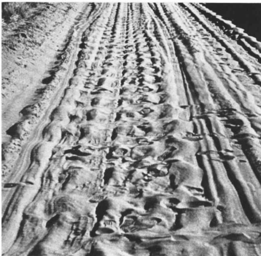
DEEP CORRUGATIONS were formed in this sandy road in the dry uplands of Australia's Northern Territory. They are most pronounced in the unpacked sand between the major ruts.
