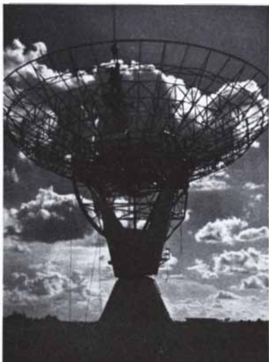
Shown under construction is 85 foot Az/E1 antenna designed and built by Rohr for Radiation Corporation for Atlantic Missile Range
