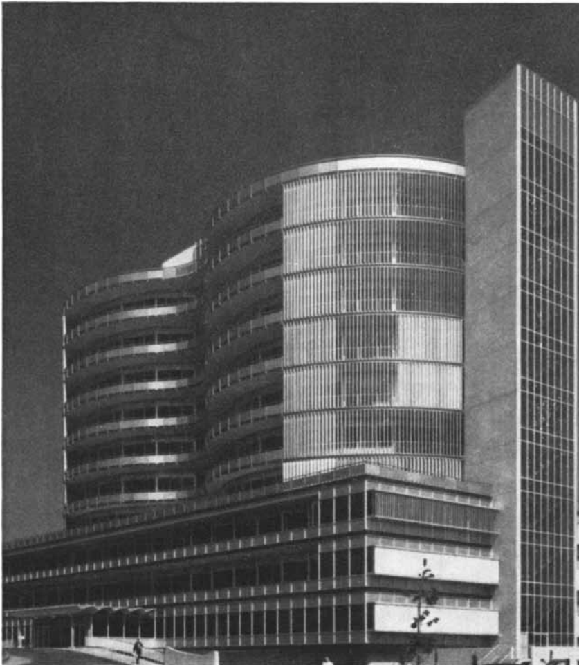
MODERN HOSPITAL , controversial in some respects, was built by the Kaiser Foundation at Panorama City in San Fernando Valley of California. It has 133 beds and is a medical center as well, providing care for 60,000 members of prepaid, group-practice medical-care plan. Rectangular three-story base has medical offices and diagnostic facilities. Twin seven-floor, circular columns above hold the hospital. Stair wells are at the ends of the columns. Several other circular hospitals have been built previously in various parts of the country.
