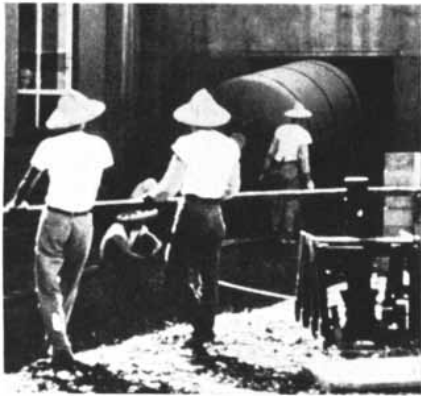
Van de Graaff accelerator being installed
