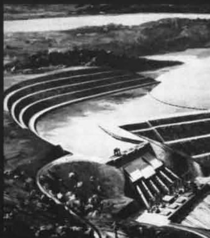
IN GHANA. The Volta River project—major hydroelectric development to electrify most of Ghana—has economic support in Volta Aluminium Company, Ltd., the nation's first major power customer, first primary aluminum producer (Kaiser Aluminum sponsored).
