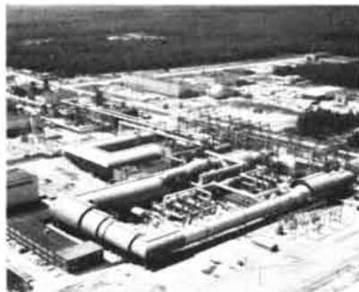
Propulsion Wind Tunnel and other facilities at Arnold Engineering Development Center.
