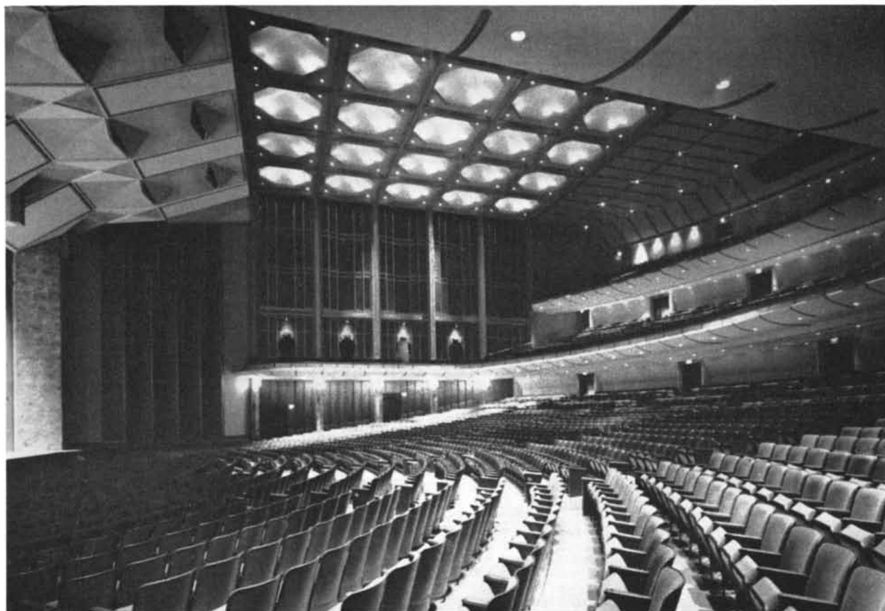
SEATTLE OPERA HOUSE has many acoustical features. Rear walls at all levels are inclined forward to prevent echoes and reflect sound beneficially. Wood panels on side walls can be opened to
