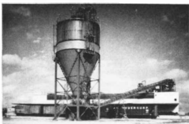
Unloading operations to this carbon black storage tank are precisely controlled by the Toledo Scale Automatic System.
