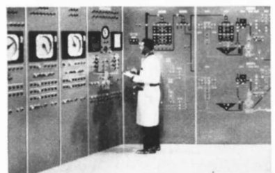
All controls are in self-contained "modules" for ease of expansion. Additional modules can be added, and locked into the Banbury control.
