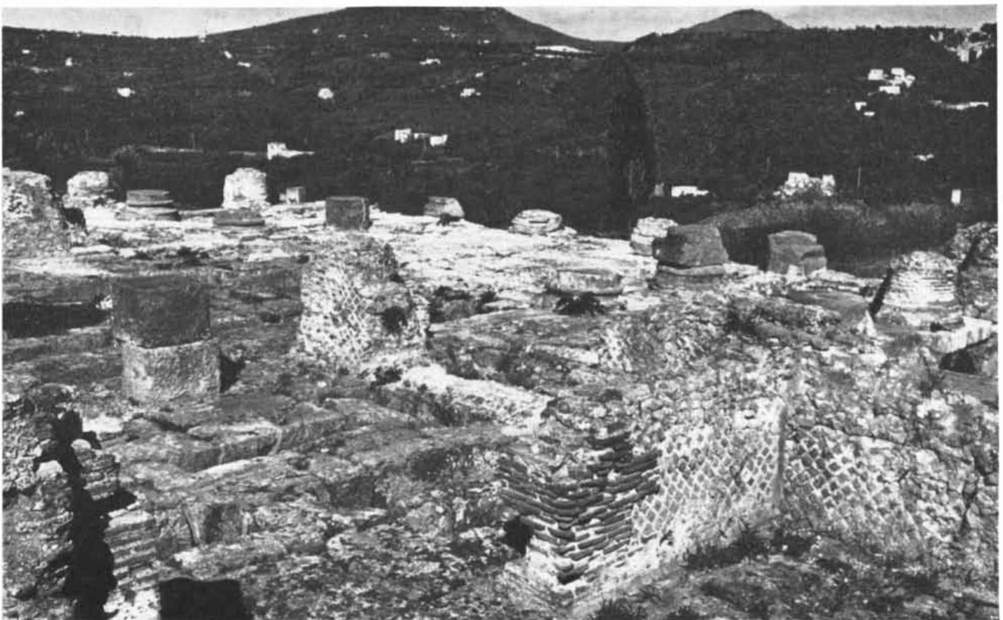
RUINS OF TEMPLE OF APOLLO on Cumae's acropolis reveal some of the differences between Greek and Roman construction methods. The large limestone blocks are from the Greek temple
