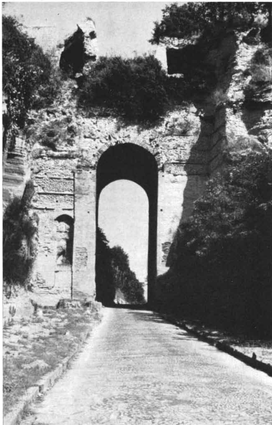
ARCUS FELIX was built about A.D. 95 to provide a more direct route through Mount Grillus between Cumae and Naples. The road under the arch is paved with its original stone.
