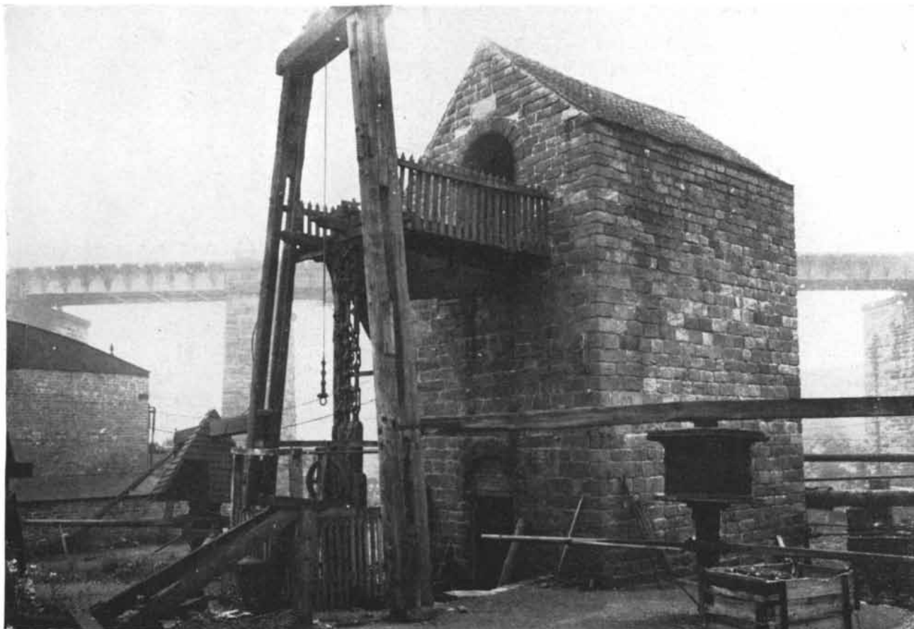
WORKING PUMP of Newcomen design is shown at a colliery in England. The pump was in use from 1791 until 1918. Subsequently
