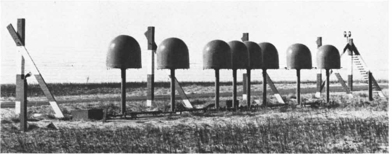
LOCALIZER-BEAM ANTENNAS of the Instrument Landing System send out radio signal in line with center of runway. These
