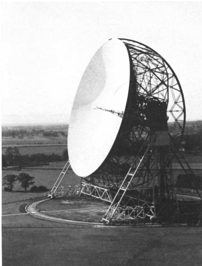
THE 250-FOOT TELESCOPE at Jodrell Bank is the largest fully steerable antenna in the world. It was used to make many of the important new observations discussed in this article.
