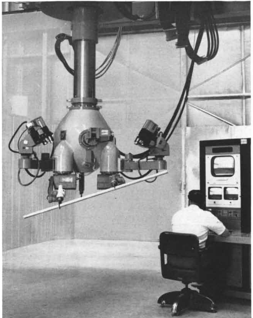
UNILATERAL MANIPULATOR responds to commands from an operator who closes separate circuits for each motion. Such systems are controlled by vision only. This is Minotaur I, built by General Mills for maintenance of a reactor at Los Alamos Scientific Laboratory.
