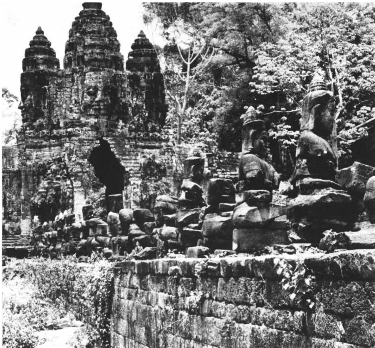
LATERITE CONSTRUCTION appears in the temple of Angkor Wat near Angkor Thom, a major city of the ancient Khmer civili-
