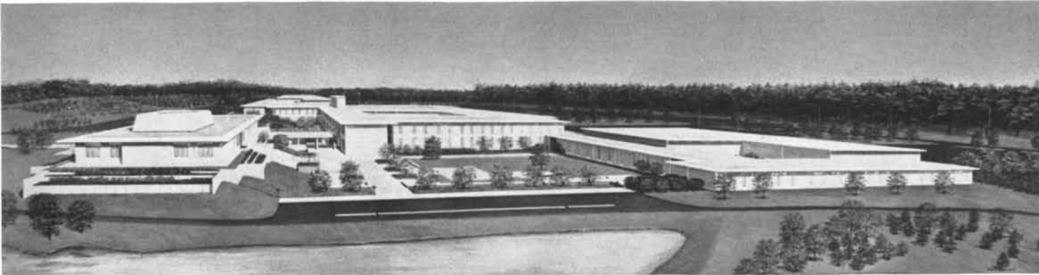
Lockheed-Georgia Research Center Now Under Construction
