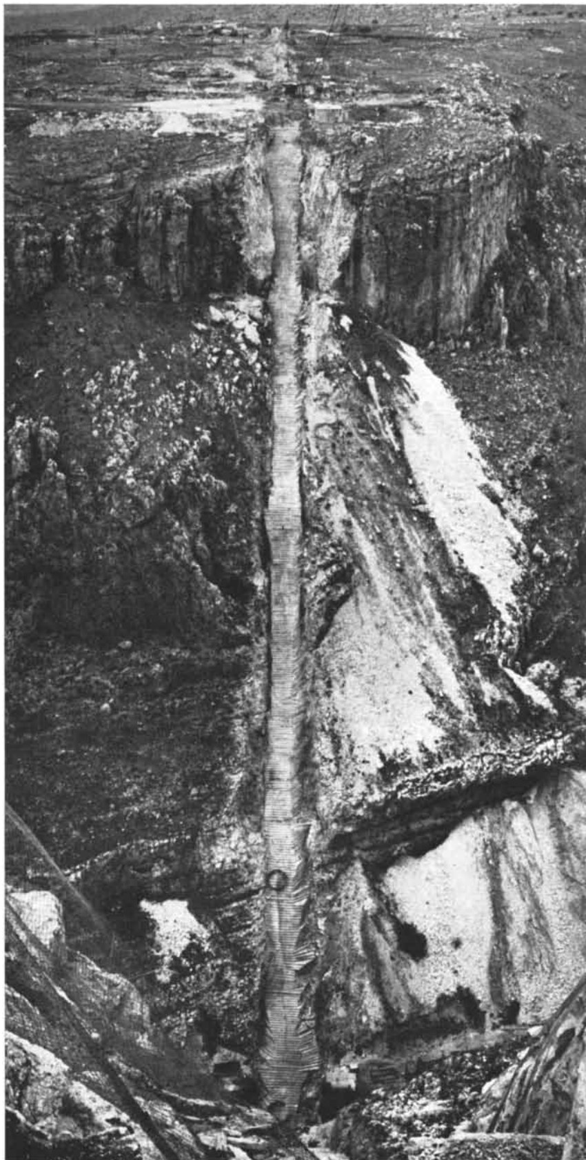
“INVERTED SIPHON” carries the trunk line of Israel’s water project down to a deep wadi, under the bed of the wadi and up the other side. In spite of its name it has no siphoning action but instead carries water by contained fall on the down side and by the resulting force on the up side. “Inverted” means that the apex of the structure is at the bottom.
