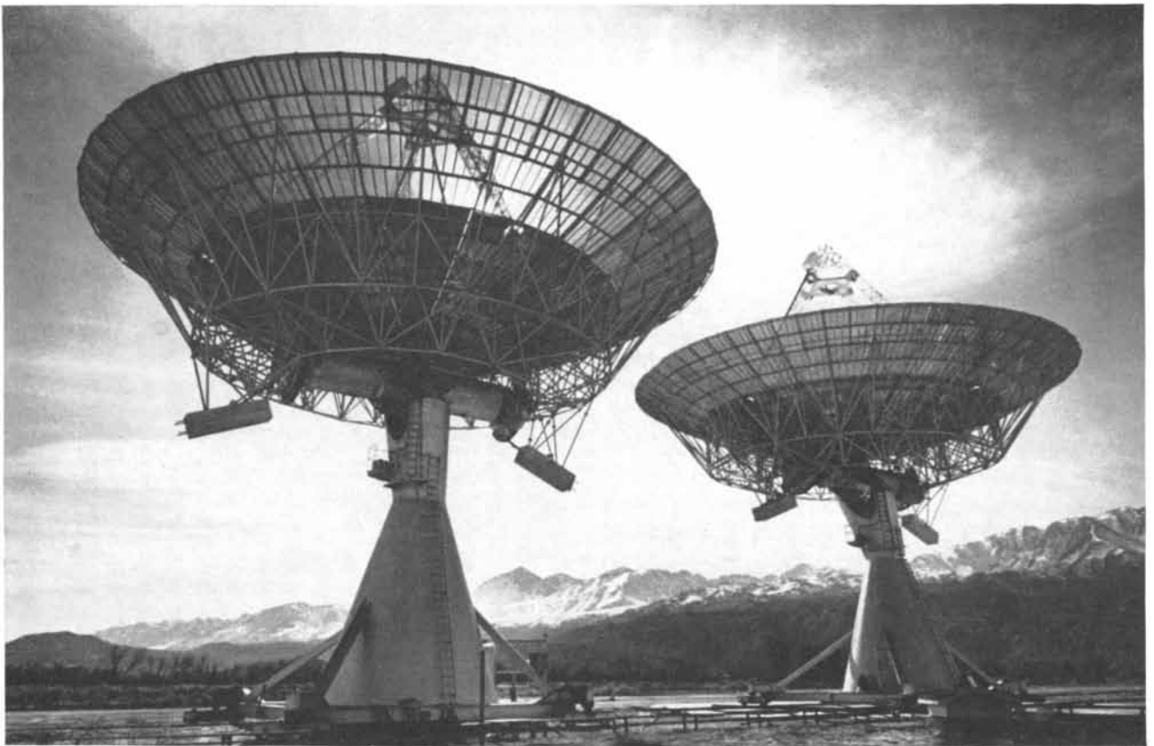
TWIN RADIO TELESCOPES , 90 feet in diameter, are the chief instruments of the Owens Valley Radio Observatory operated by the California Institute of Technology. The telescopes can be
