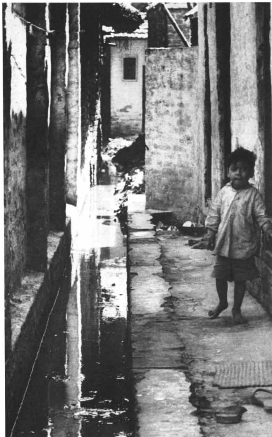
OPEN SEWER runs along one side of a narrow slum street in Calcutta. Such methods for the disposal of human wastes, together with the slum dwellers' general use of untreated water for cooking and drinking, has made the city the center of endemic cholera in India.
