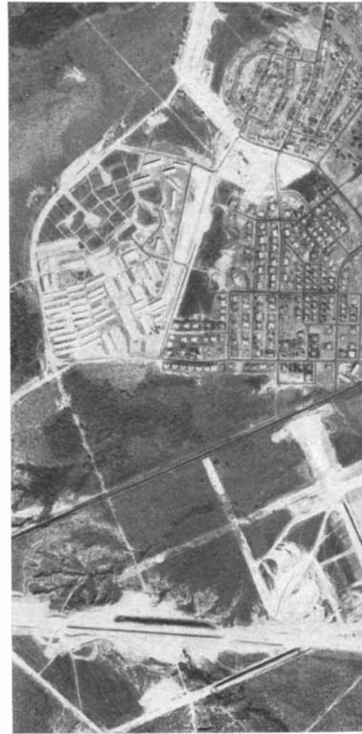
EXISTING COMMUNITIES on the site of the future Ciudad Guayana are seen in this
