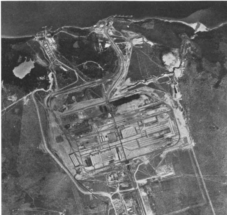
STEEL MILL , built by the Venezuelan government, is now in operation. The mill will be the nucleus of the heavy-industry complex planned for the western end of the new metropolis.
