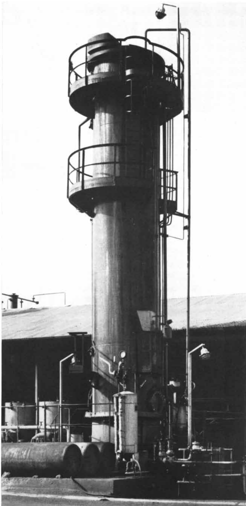
LARGE PILOT PLANT at the Lavera refinery is now producing protein from petroleum on a scale permitting engineering studies. With an outlay of some 40 million tons of petroleum the world's refineries could produce 20 million tons of pure protein per year.
