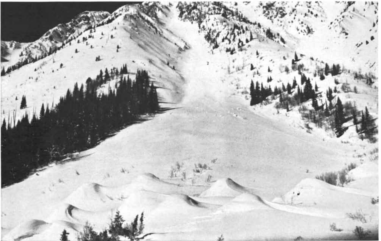
BREAKER MOUNDS serve to impede avalanches near the Trans-Canada Highway in British Columbia. Austrian engineers discovered the mound technique when they left heaps of rubble from
