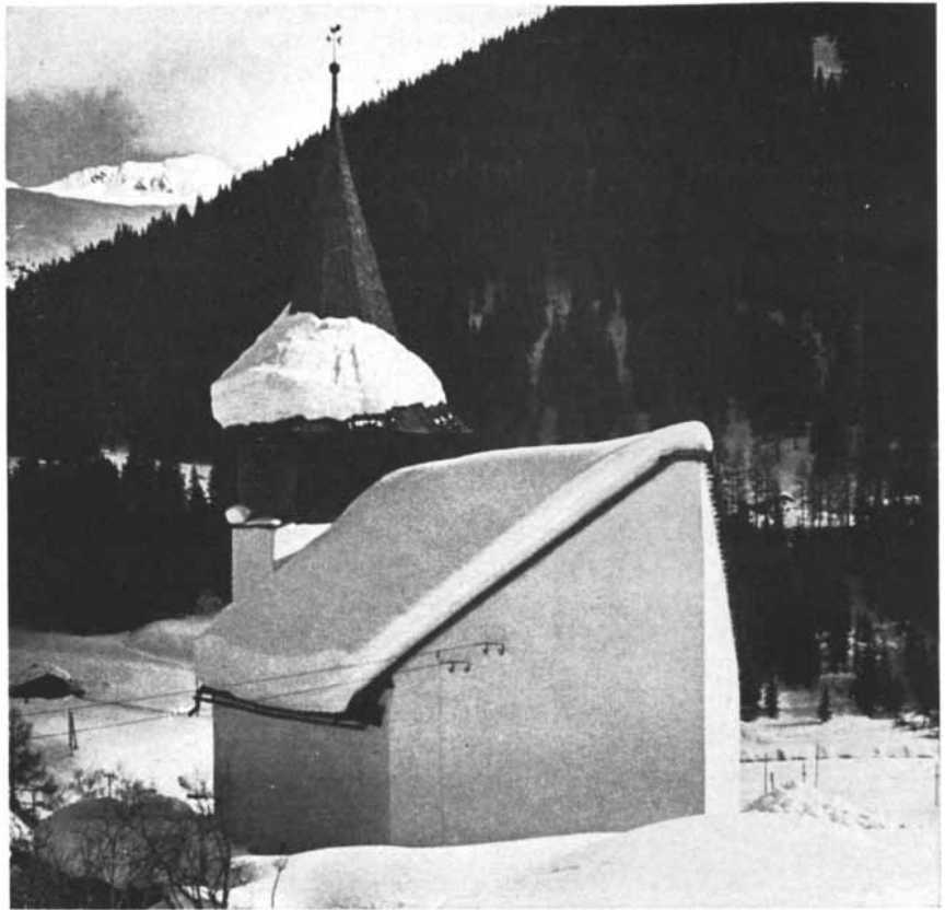
WEDGE TECHNIQUE , long in use in the Alps, involves incorporating a wedge on the uphill side of a building, as on this church near Davos, to divert a flowing mass of snow.
