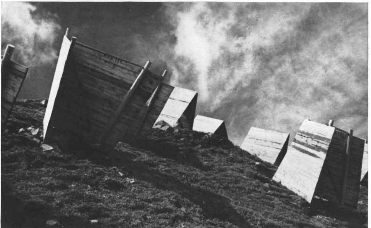
WIND BAFFLES constitute another experimental array in Switzerland. They were built to create an irregular flow of wind in an area
