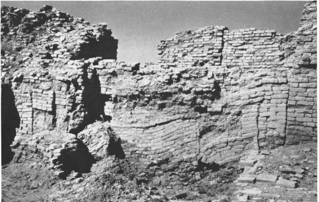
FLOOD DAMAGE at Mohenjo-daro is evidenced by slumping brick masonry ( center ), which presumably reflects erosion of the city's
