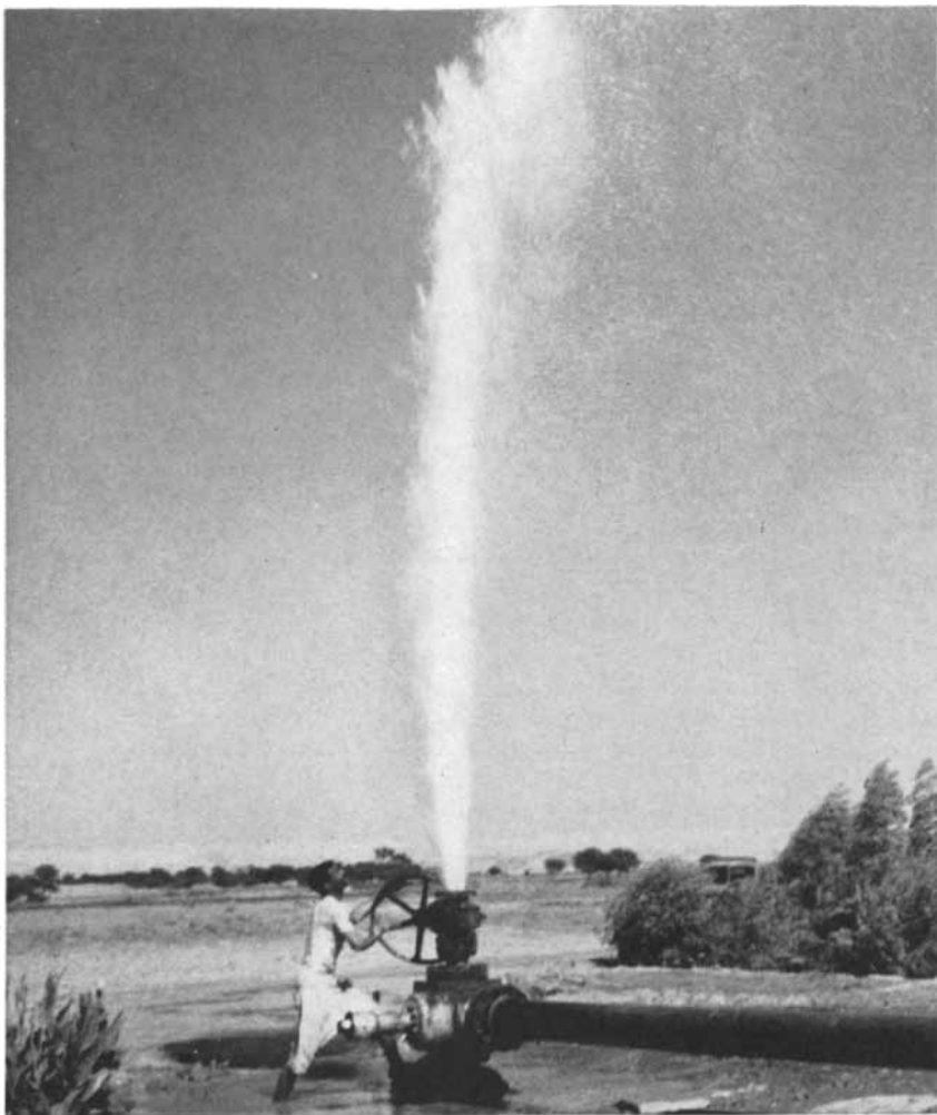
ARTESIAN WELL spouts water high above the desert in the United Arab Republic's New Valley project. The project involves the drilling of more than 200 boreholes, each several hundred yards deep, into a sandstone aquifer to produce water for making the desert fertile.
