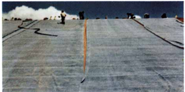
After the rubber is allowed to "relax", the edges are overlapped and bonded together with adhesive.
