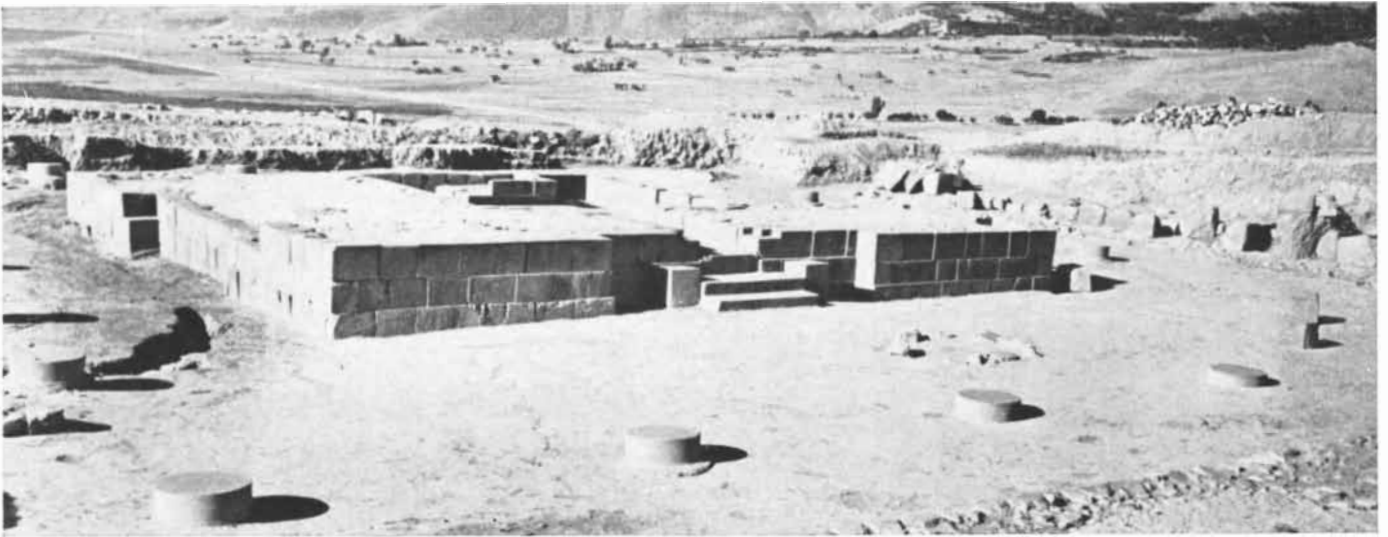
STONE FOUNDATION of the temple shrine at Altintepe consists of three masonry courses on top of which the Urartian builders
