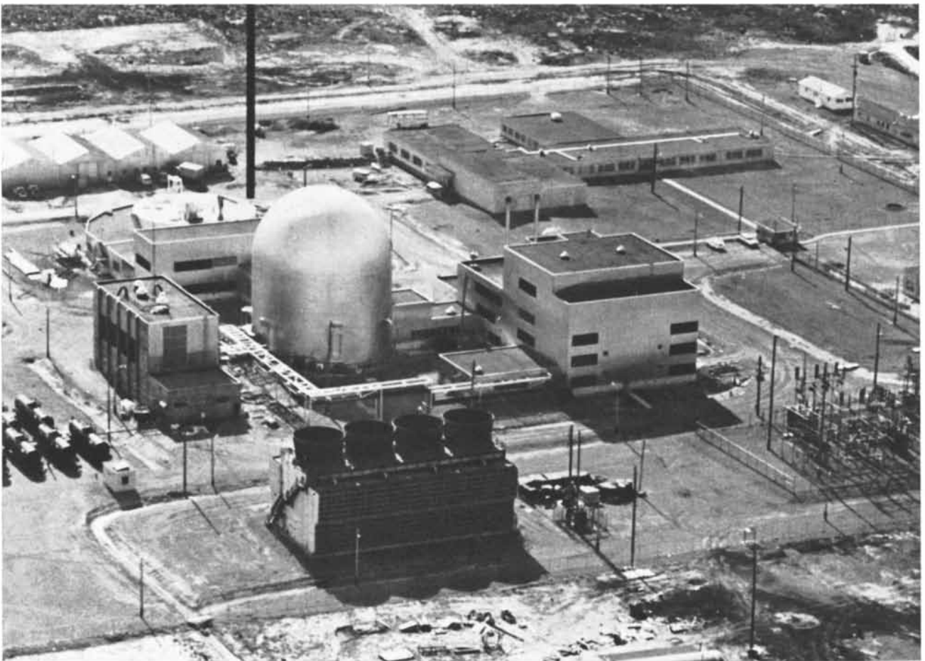
SECOND-GENERATION BREEDER REACTOR is in the domed structure. In the foreground are cooling towers; at left is a sodium-boiler plant; behind the domed structure is a fuel-reprocessing
