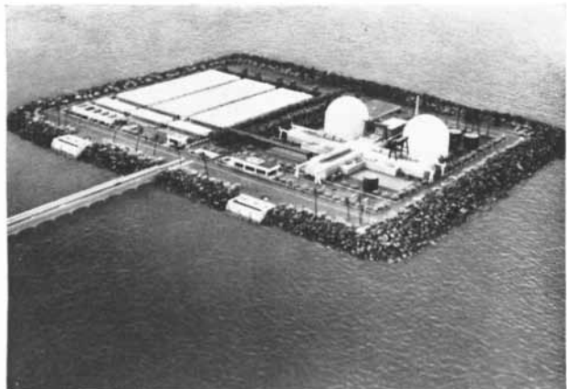
From the sea. Bendix oceanographic studies are helping in the conceptual design and location of the world's first large-scale sea water conversion plant to use nuclear power. This dual-purpose structure, to be built on a man-made island off southern California, will supply enough water for a city the size of San Francisco and more power than Hoover Dam.
