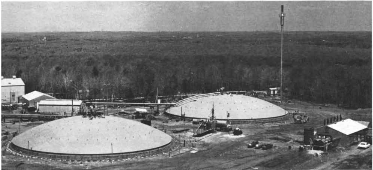
FINISHED TANKS at the Hopkinton plant looked like this when double-walled steel roofs were built over the pits shown in the photograph at the top of this page.
