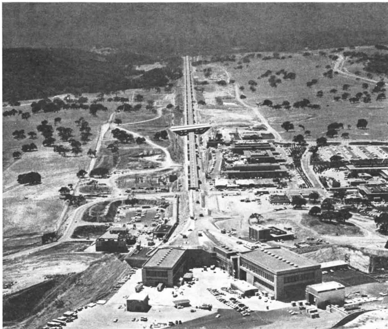
TWO-MILE ACCELERATOR is seen from the air. The long structure resembling a highway houses the accelerator tunnel. In the foreground are the two target buildings, into which the 20-billion-
