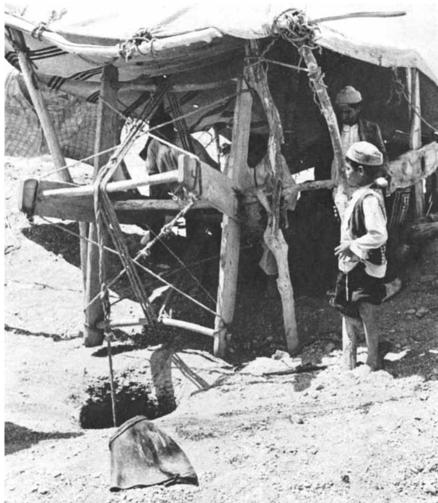
WINDLASS CREW , sheltered from the sun by an improvised tent, raises a load of accumulated silt in the process of cleaning a qanat conduit tunnel. Standing beside the tent is a child who is needed on this job because the ventilation shafts are smaller than usual.
