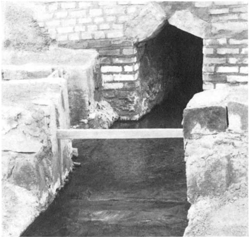
MASONRY MOUTH of an Iranian qanat is equipped with a pair of sluice gates that allow diversion of the water into separate canal systems. The amount of qanat water that may be allotted to village or individual is sometimes determined by decisions made centuries ago.
