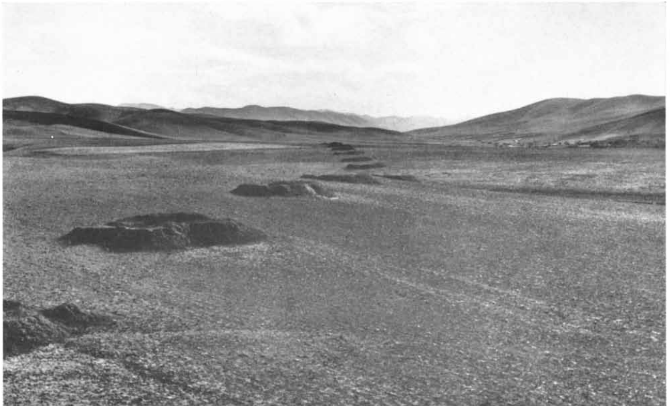
ROW OF CRATERS , each one marking the mouth of a qanat ventilation shaft, runs across an arid plain in western Iran. The walls
