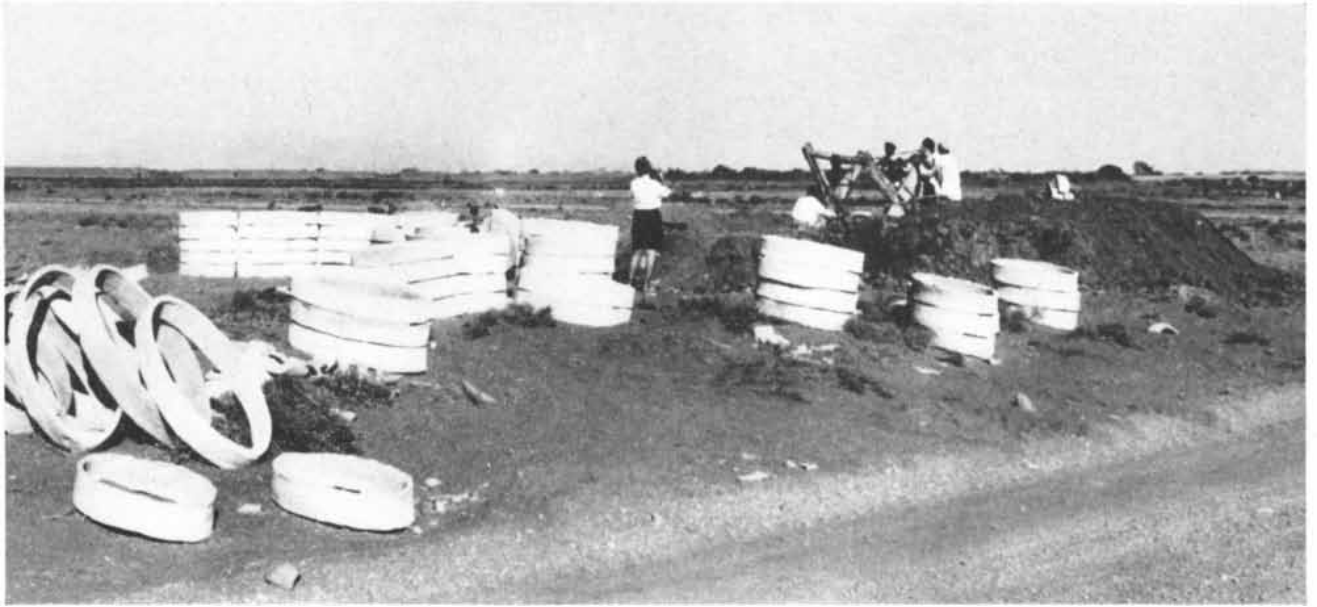
TILE HOOPS are piled up near one of the vertical shafts that lead to the conduit tunnel of a qanat under construction in rural
