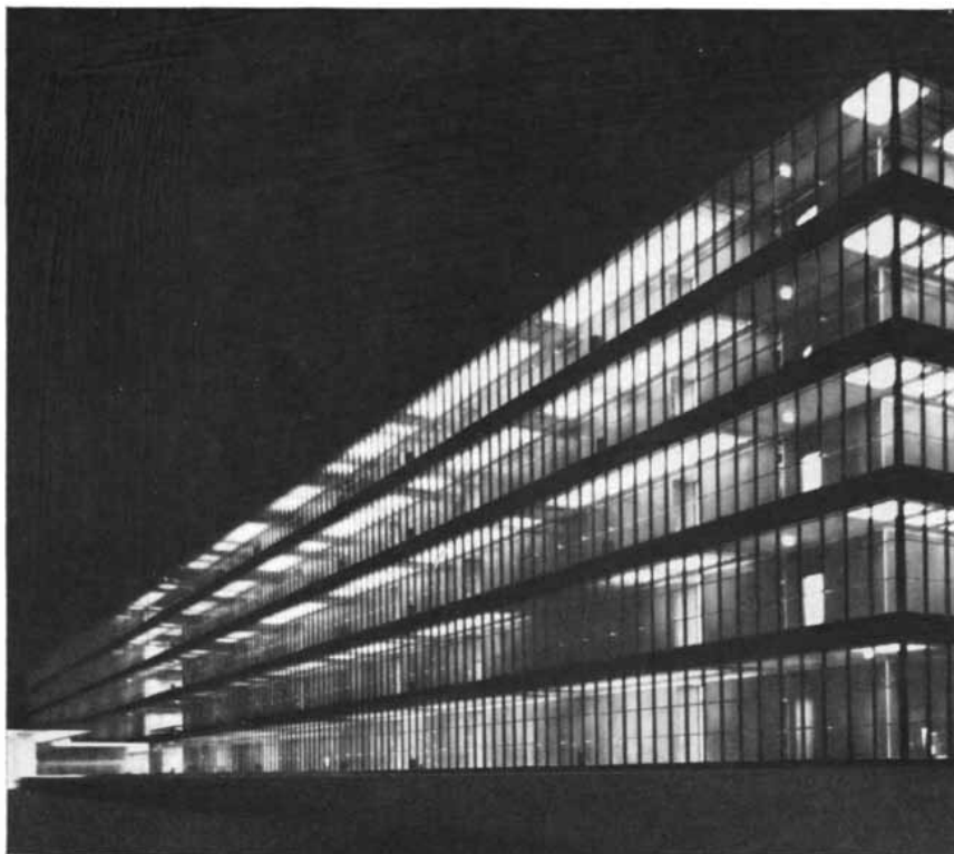
TRANSPARENT BY NIGHT , the Holmdel building emits a glow of light once the level of exterior illumination falls below that of the interior. The interior walls are now mirrors to the occupants. The glass rejects nearly 80 percent of the solar heat load. It is made by the Kinney Division of the New York Air Brake Co. Architects were Eero Saarinen and Associates.
