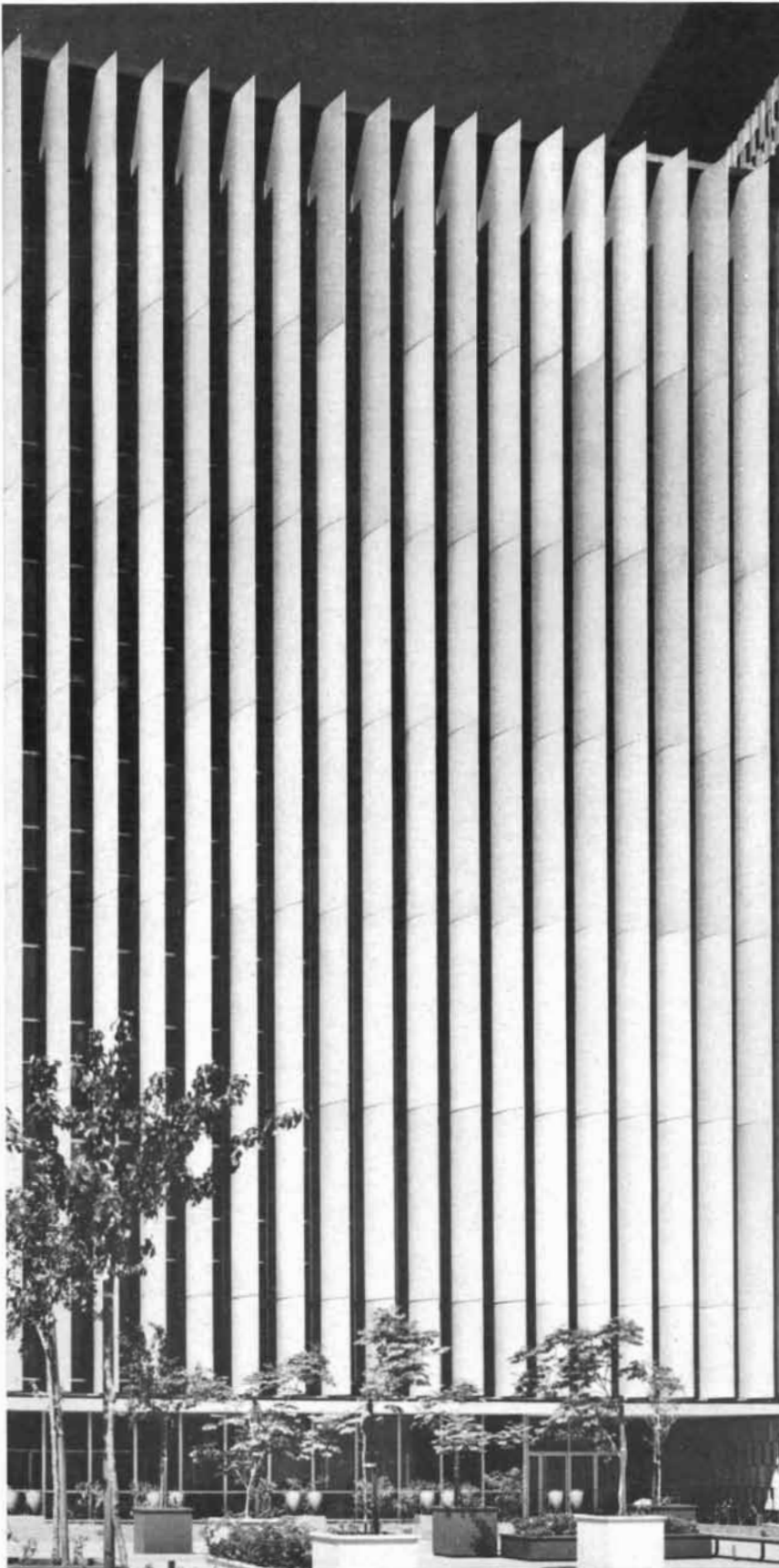
CONTROL OF LIGHT AND HEAT is achieved at the Los Angeles Hall of Records by vertical louvers that resemble a venetian blind turned sideways. The angle at which the louvers are set is adjusted monthly to provide maximum shade throughout the year. Architects were Neutra and Alexander, Honnold and Rex, H. C. Light and James R. Friend.
