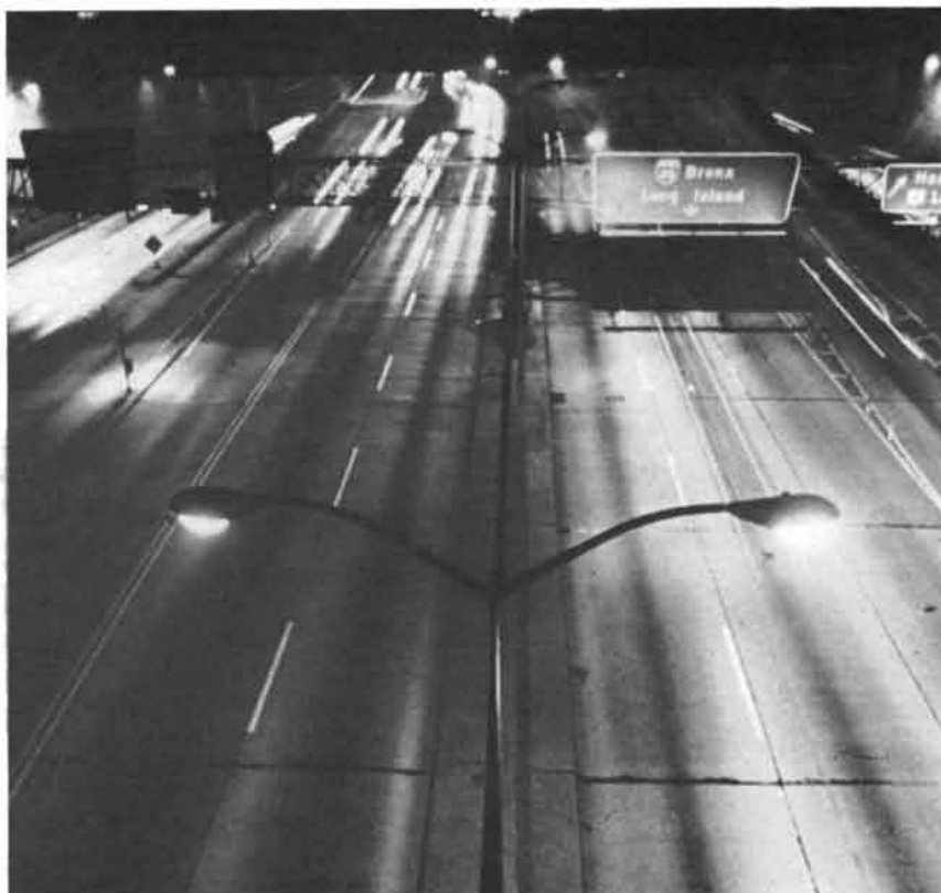
NIGHT LIGHTING of New York's George Washington Bridge shows contrast between the illumination from mercury and sodium high-intensity lamps. When the photograph was made, lamp standards over outbound lanes ( left ) contained 400-watt mercury-vapor lamps and those over inbound lanes ( right ) 400-watt sodium-vapor lamps. The illumination of the inbound lanes is two to three times brighter than the illumination of the outbound lanes.
