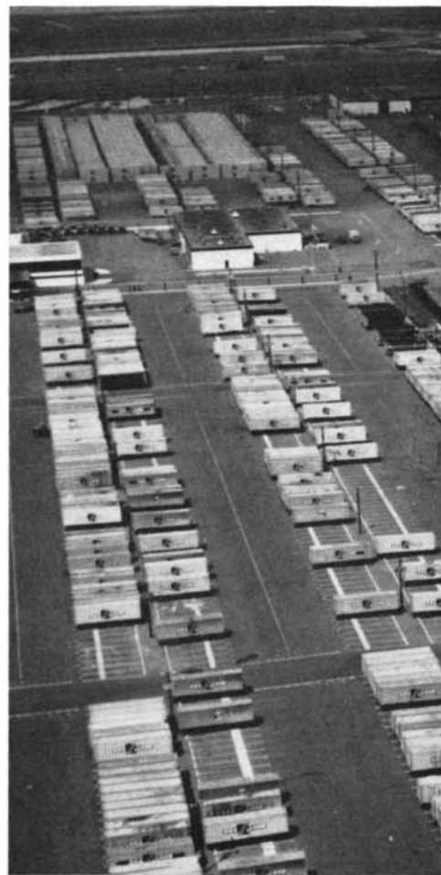
CONTAINER-SHIP TERMINAL at Elizabeth, N.J., was built by the Port of New York Authority to facilitate the movement
