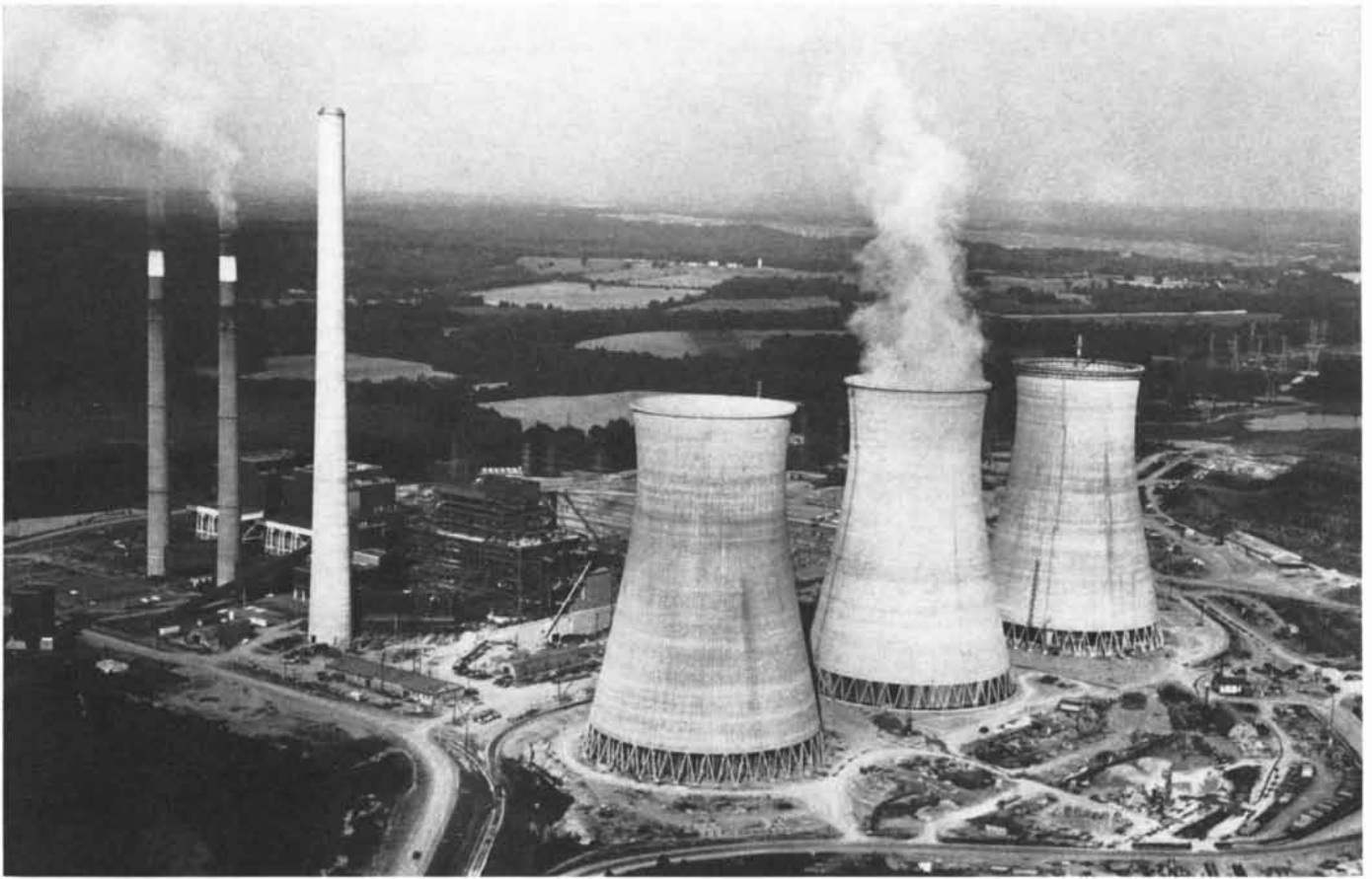
POWER PLANT being completed by the Tennessee Valley Authority on the Green River in Kentucky will be the world's largest coal-fueled electric plant. Its three wet, natural-draft cooling towers,
