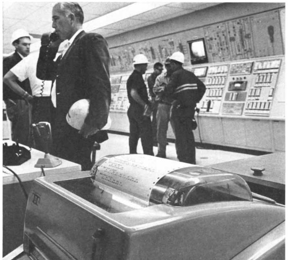
CONTROL ROOM at the Torrance refinery includes the printer in the foreground, which provides a computer print-out of the chromatographic analyses of the 27 process streams.
