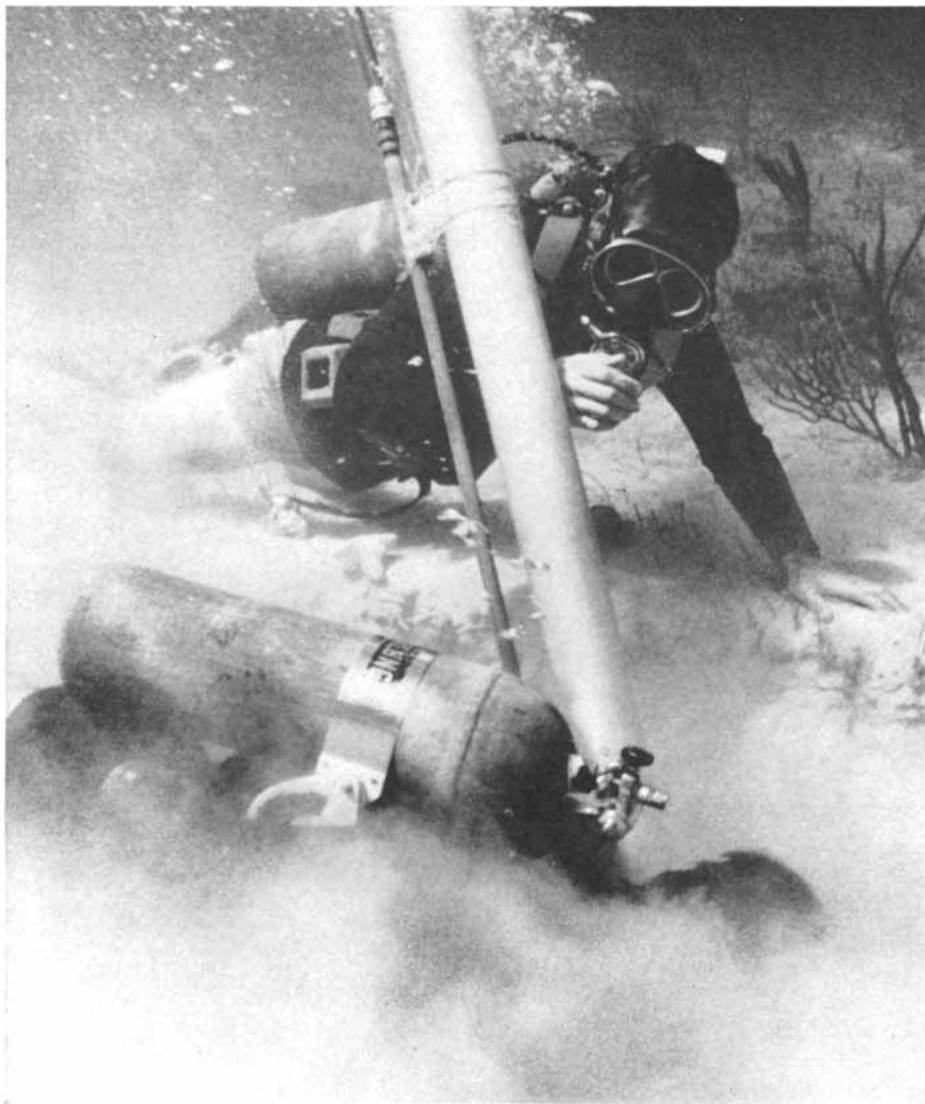
DIVING GEOLOGISTS of the Shell Oil Company probe the ocean floor at a depth of about 20 feet on the Bahama Banks. The pipe and hose slanting across the center are parts of an air-lift apparatus that they are using to obtain information helpful in the search for oil.
