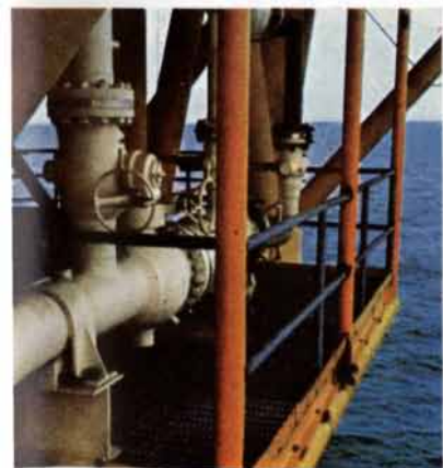
Cameron ball valves and operators for offshore platforms and underwater pipelines.
