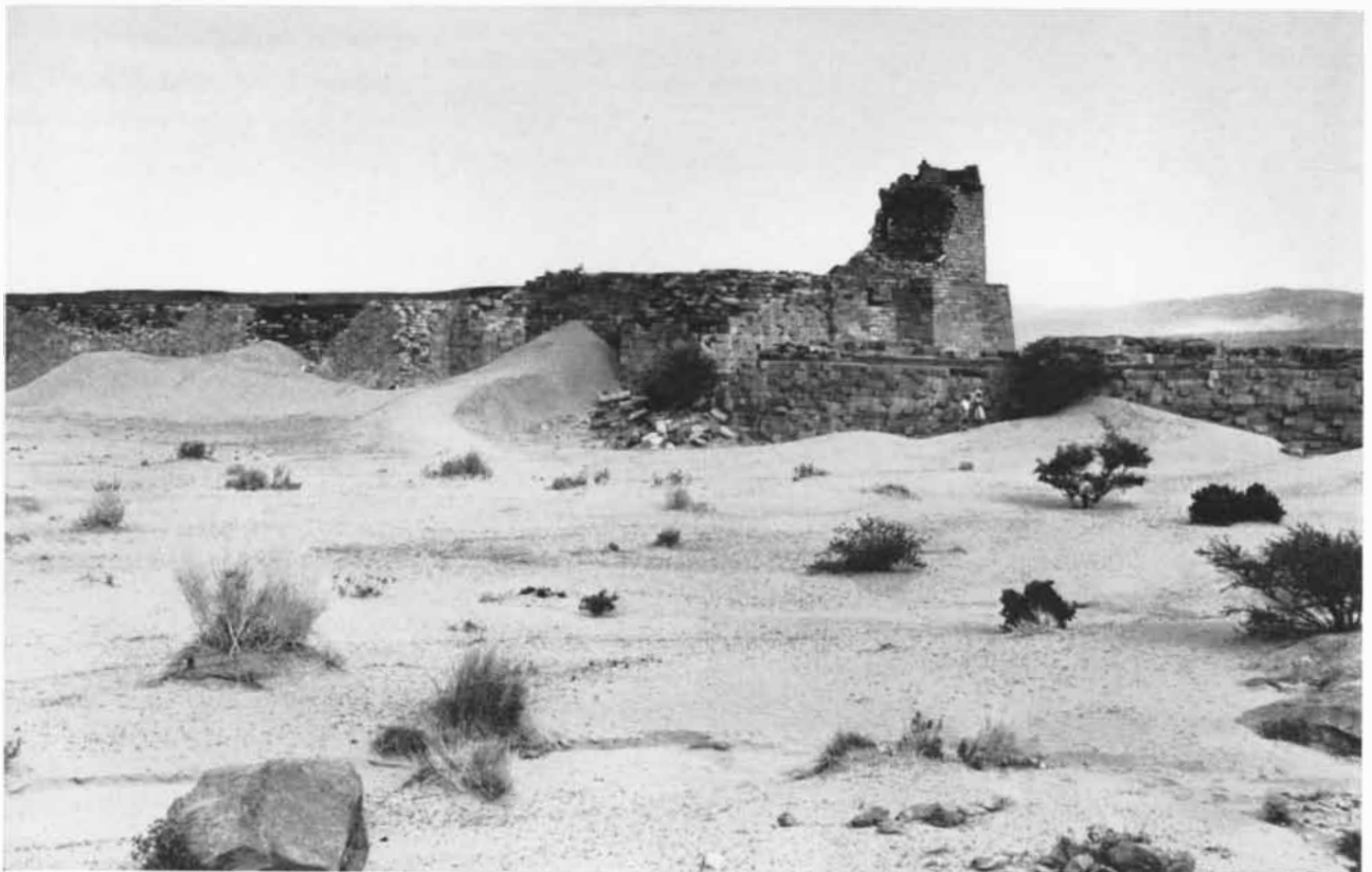
NORTH SLUICE of the Marib dam is seen from the west. The dam itself was built of earth that was faced with stone. It ran some
