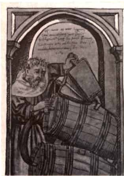
COMPRESSED AIR is serving as a propellant, forcing wine through a tube from one barrel to another, in a painting made in Nuremberg in A.D. 1474. Large-scale movements of materials with compressed air had to await the development of better blowers.
