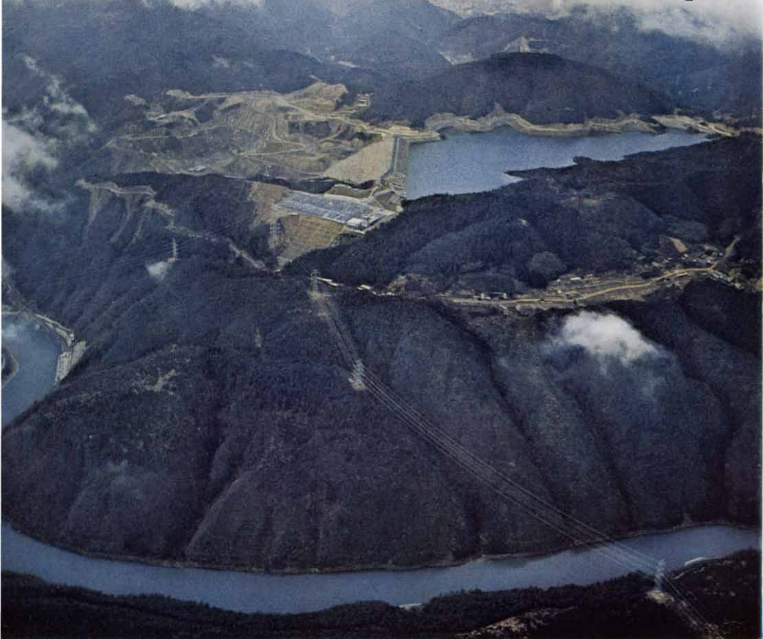
Bird's-eye view of Kisenyama Power Station site near Kyoto, Japan where Hitachi's 322,000 HP pump-turbine is now in operation
