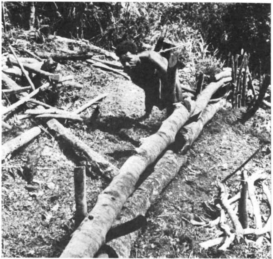
FENCE-BUILDING is one of the more energy-consuming tasks in preparing a garden. Fences must be pig-proof to keep out both domestic swine and feral swine from the forest.
