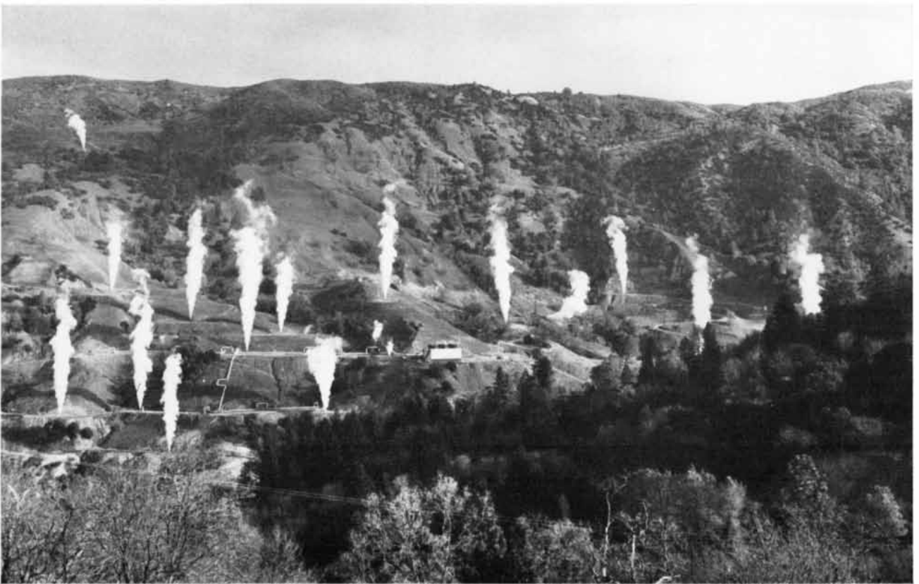
STEAM WELLS tap geothermal energy for the production of power at a plant operated by the Pacific Gas and Electric Company at
