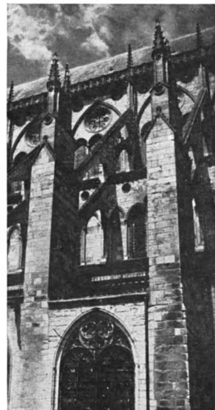
ing buttresses also come closer to the roof. The piers at the choir are seen to be reinforced, just above their intersection with the flying buttresses, by the parapet: the wall just below the roof ( right ).
