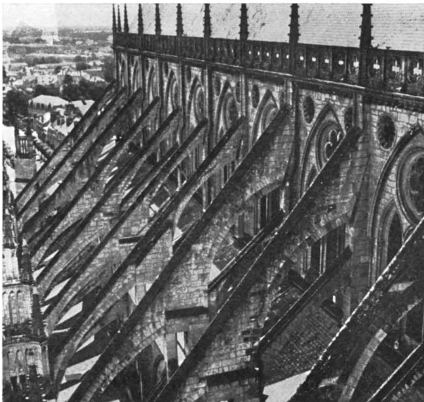
FLYING BUTTRESSES of Bourges ( left ) were built at different times. Those supporting the choir ( background ) are lighter than those used for the nave, which was constructed later; the nave fly-
