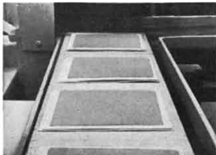
1500° C furnace was specially designed to fire these new substrates. The relatively low temperature results in smooth substrate surfaces for practically fault-free thin film bonding.
