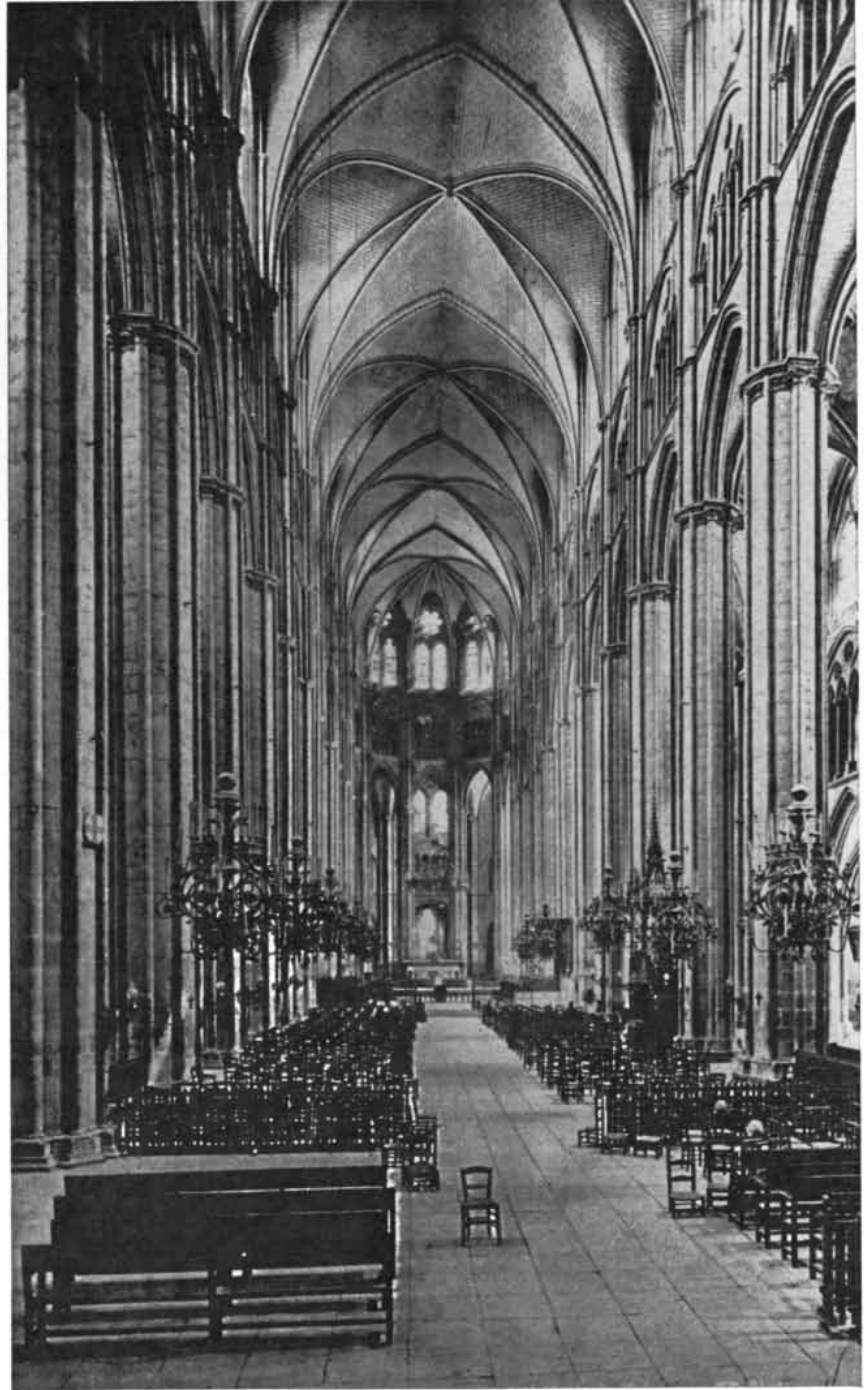
MAIN VAULTING of Bourges rises 120 feet above the floor. Whereas the vaulting of Chartres and almost all other High Gothic cathedrals is quadripartite (see illustration on page 92), Bourges's vaulting is sexpartite. Alternate piers meet one vault rib or three ribs.
