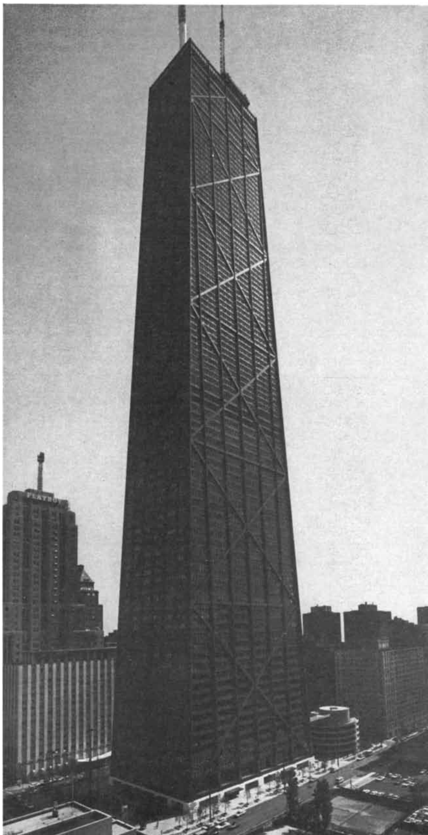
EXTERIOR FRAMEWORK of immense steel members sustains all wind loads in the 100-story John Hancock Center in Chicago. On each face of the building the braces form X trusses over five panels of 18 stories each and a K truss over the top 10 stories. The tower is a braced, tubular cantilever, a skyscraper counterpart of the 19th-century iron bridge bent. Bending forces induced by the wind are removed from the interior frame and confined to the trussed walls. In addition any pattern of vertical loads is distributed equally among the columns. Architects and engineers were the Chicago office of Skidmore, Owings & Merrill.
