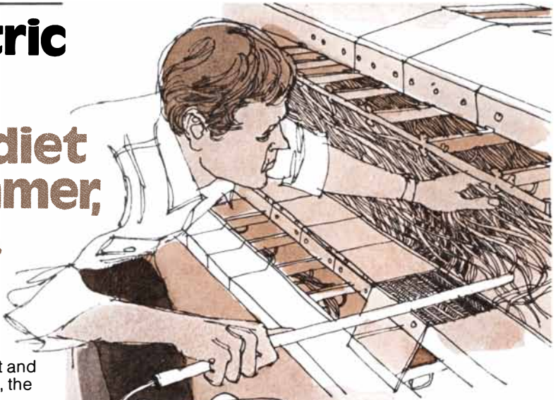
Central office distributing frame. Reach in, pull out an old wire, and solder in a new one.
