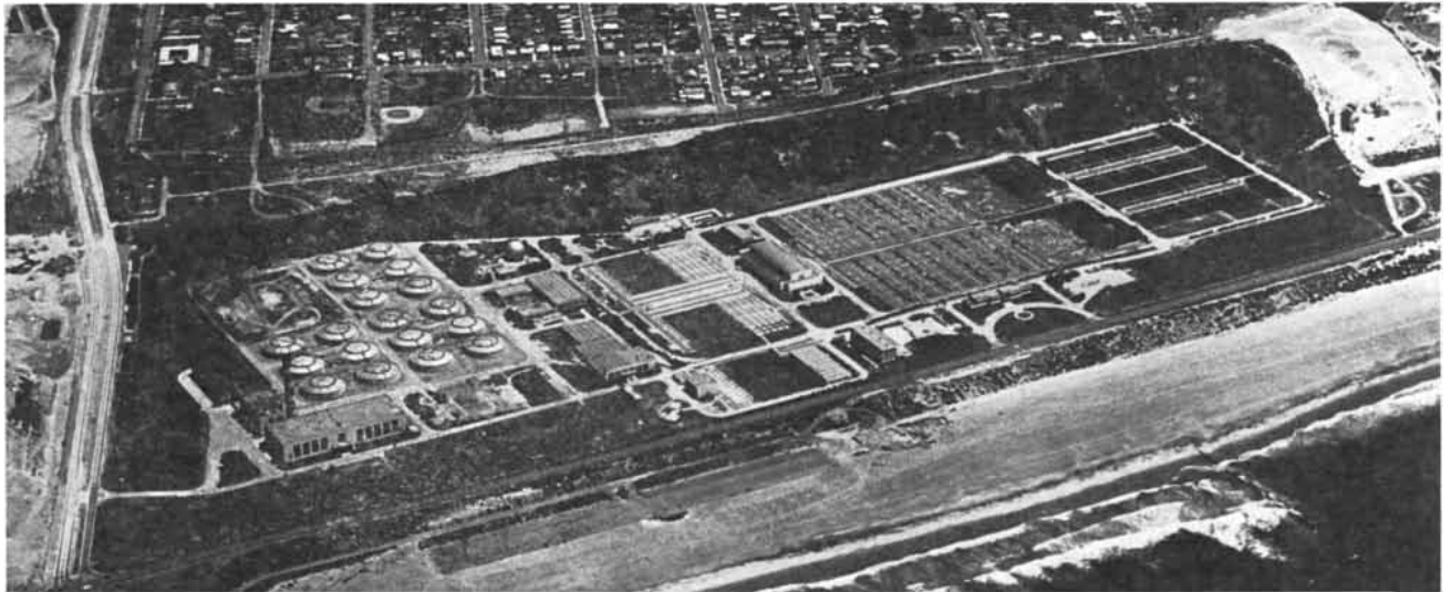
SEWAGE-TREATMENT PLANT serves the City of Los Angeles, discharging into the Pacific Ocean about 235 million gallons per day of primary treated effluent and 100 million gallons per day of secondary effluent. The discharge pipe is 12 feet in diameter and
