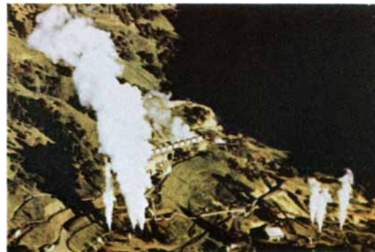
The geothermal plant can use a natural steam field, like The Geysers, near San Francisco, which will generate a half million kilowatts this year. The earth's heat can also be tapped by forcing cold water miles down onto hot rocks. Our Western states have many geothermal areas which could provide considerable power in the future.
