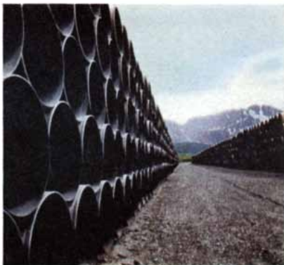
It took over one-half million tons of steel to make the 798 miles of pipe for the project. The sections are 40' and 60' long, 48" in diameter.
