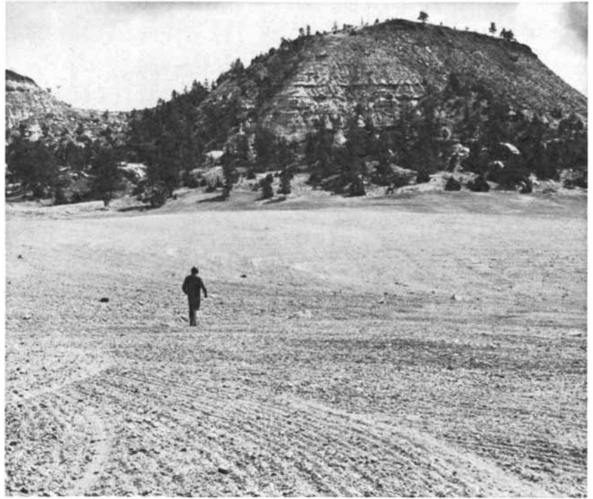
RECLAMATION OF STRIP MINE is in progress at the Big Sky Mine of the Peabody Coal Company in Montana. Here the spoil banks have been shaped and partly seeded with oats and alfalfa, which serve as cover crops for a mixture of native grasses. The view is southeast toward hills and coniferous trees that were not affected by the strip-mining operation.
