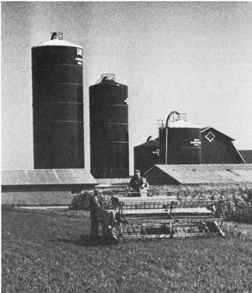
MODERN SILOS appear behind a field of alfalfa on a dairy farm in New York. They are Harvestore silos, shiny blue structures made of steel plates coated on both sides with cobalt blue glass fused to the steel by heat. The function of a silo, which may also be made of wood or concrete, is to minimize the amount of oxygen that can reach a crop and cause spoilage. When the crop has been chopped finely and put in the silo, it is pickled (and thus preserved) by the action of lactic acid bacteria that thrive in the absence of oxygen.
