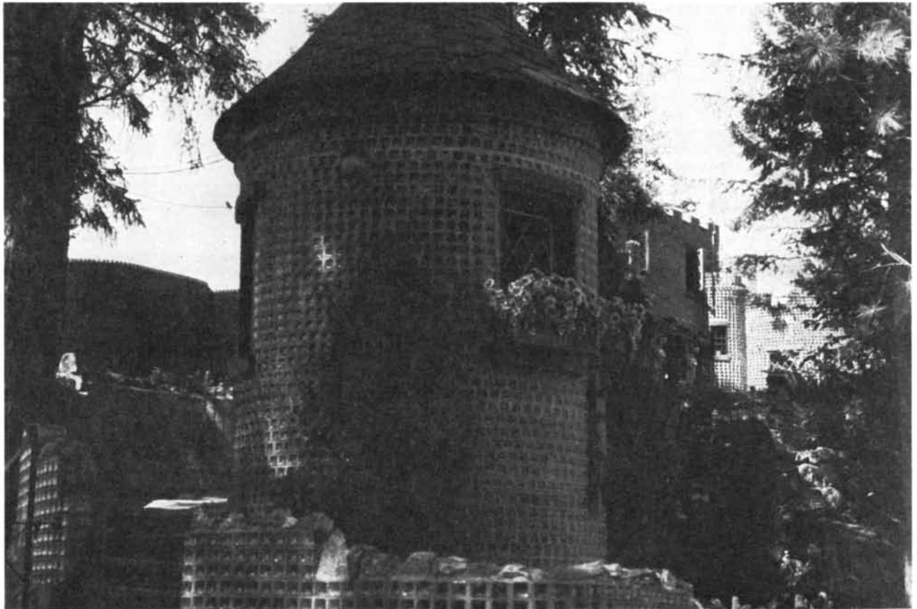
A mansion built of empty embalming-fluid bottles, from All Their Own: People and the Places They Build
