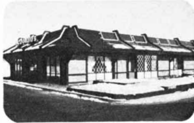
McDonalds restaurant uses Revere Sun-Aid collectors as a natural addition to the roof.
