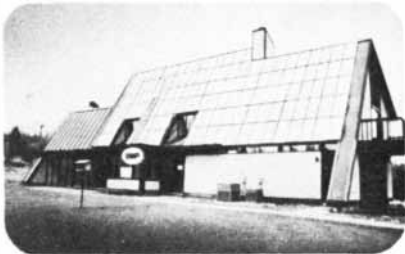
Revere Sun-Roof collectors are an integral part of the roof of this N.Y. State residence.
