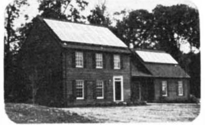
Revere modular solar collectors help reduce the fuel bills for this HUD demo house.
